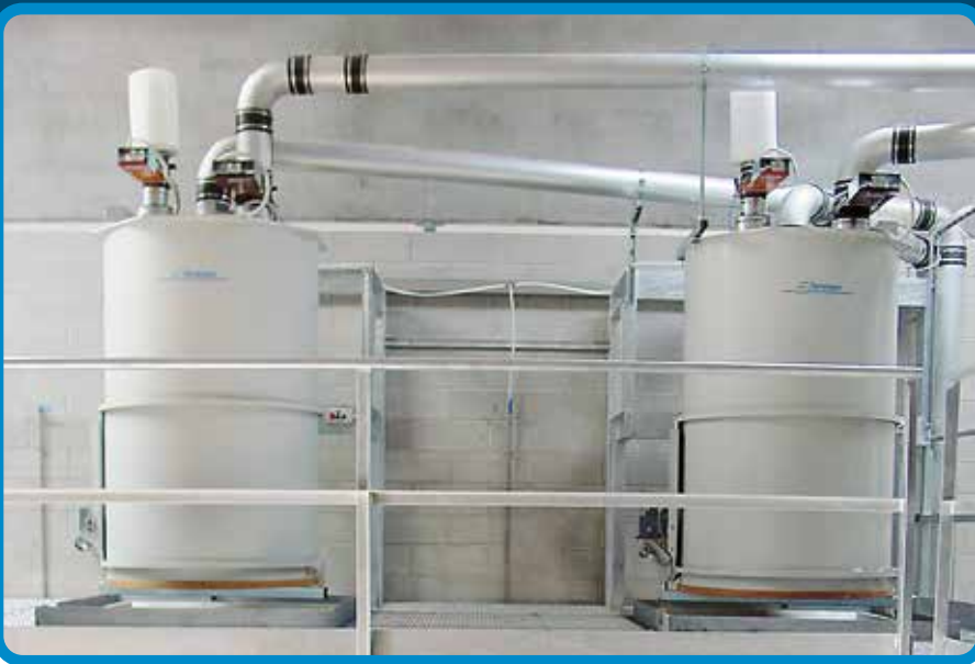
Filter system mounted on installation platform The closed-circuit system keeps your waste separate from pick-up to compaction.
