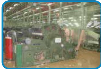
Card cleaning with compressed air (before CVS was installed).
