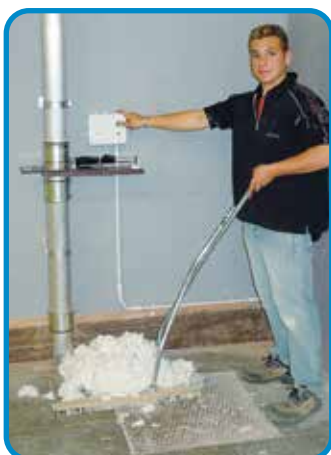
Floor sweeping: waste collected with brooms to a sweeping point
